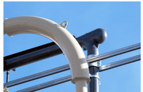
CoorsTek has replaced most of its double-wall sweep elbows (foreground) with Smart Elbow® deflection elbows (rear).
