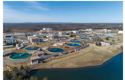
The Upper Occoquan Water Reclamation Plant supplies over 30 million gallons per day of potable water to a population of more than 300,000.
