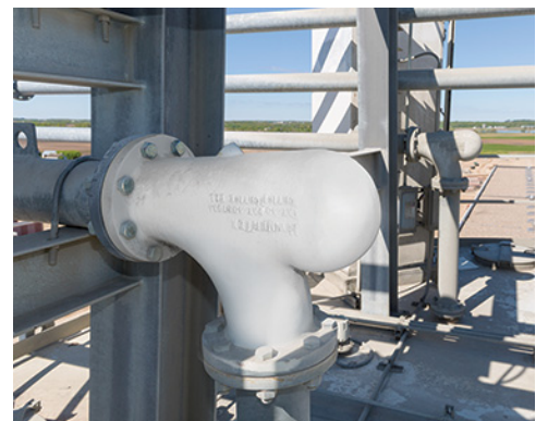
At this concrete production plant, the compact dimensions of the tight-radius Smart Elbow design minimize space requirements compared to long-sweep elbows.
